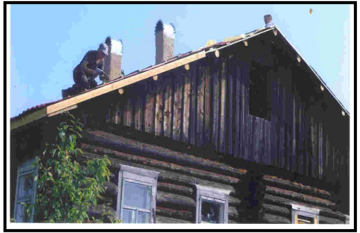
William putting some finishing touches on the the new roof.
